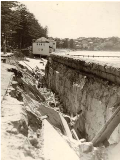
Figures 2 & 3 - Storm damage to Manly Ocean Beach seawall in 1950. The dotted line indicates original position of seawall.
