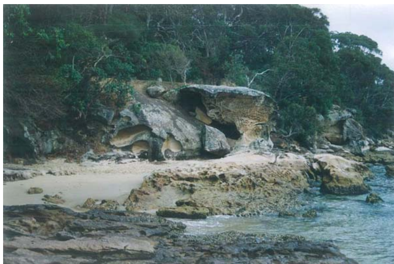
Figure 6 - Collapse of overhang feature likely. Geoheritage and cultural heritage issues have complicated the mitigation of risks yet are important considerations.
