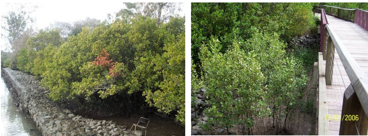
Figure 3 Rock gabions used successfully to reduce impacts of vessel wash and foreshore erosion, protecting and enhancing mangrove communities [left] and structures [right] in the Brisbane River, Queensland.
