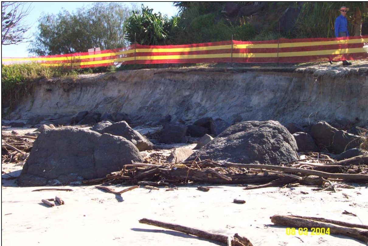
Figure 3. Erosion in the southern corner of Duranbah Beach resulting in the loss of a popular pedestrian walkway
