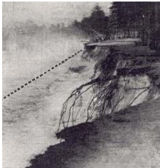
Figures 2 & 3 - Storm damage to Manly Ocean Beach seawall in 1950. The dotted line indicates original position of seawall.
