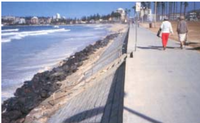
Figure 4 - Exposure of rock apron, Manly Ocean Beach in 1988
