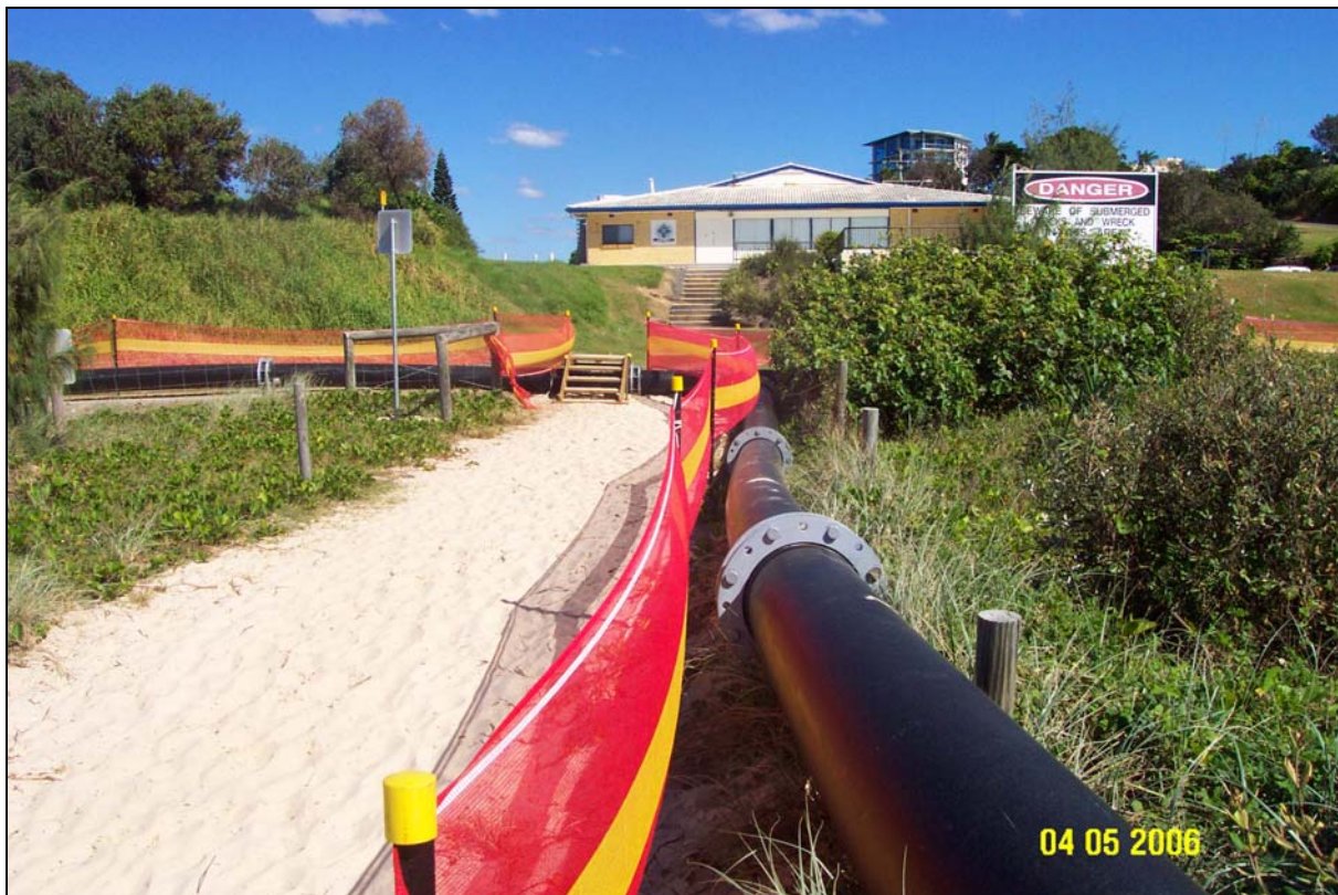
Figure 4 – Temporary pipe work and safety fencing
