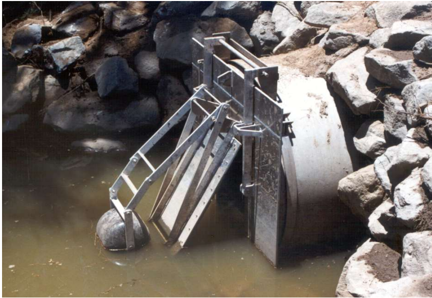
Figure 3 A typical tidally-activated gate fitted to a floodgate flap.
