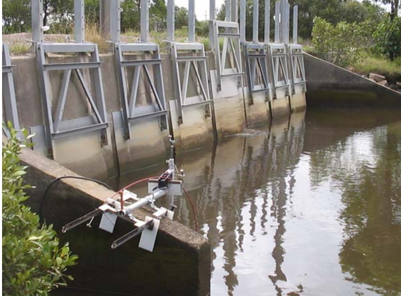
Figure 5 Eight floodgates located at Ironbark Creek draining Hexham Swamp.
