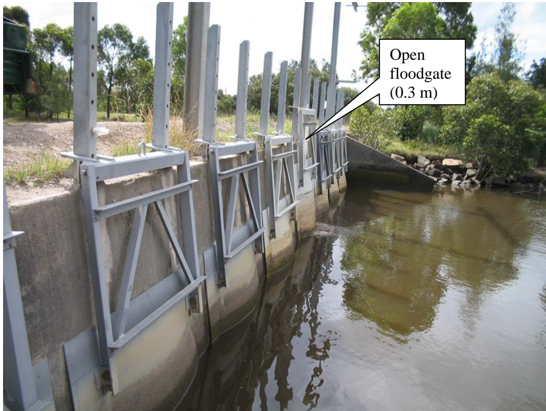
Figure 20 Floodgates at Ironbark Creek, Hunter River. Notice open floodgate at the current 0.3m level.
