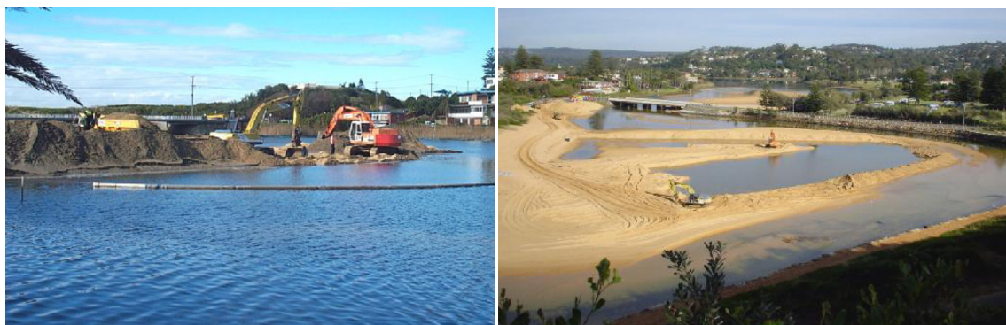
Figure 3: Dredging works in progress west (left photo) and east (right photo) of Ocean St Bridge in Narrabeen Lagoon.
