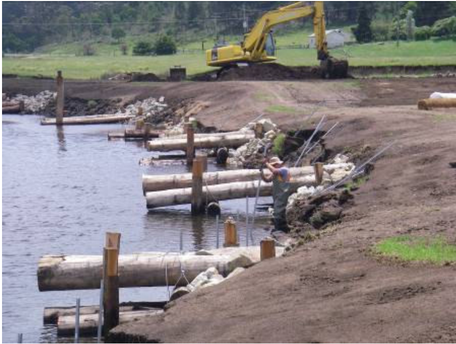
Figure 4a – Fish habitat (in foreground) and bundle groynes (in background) post installation Nov 07
