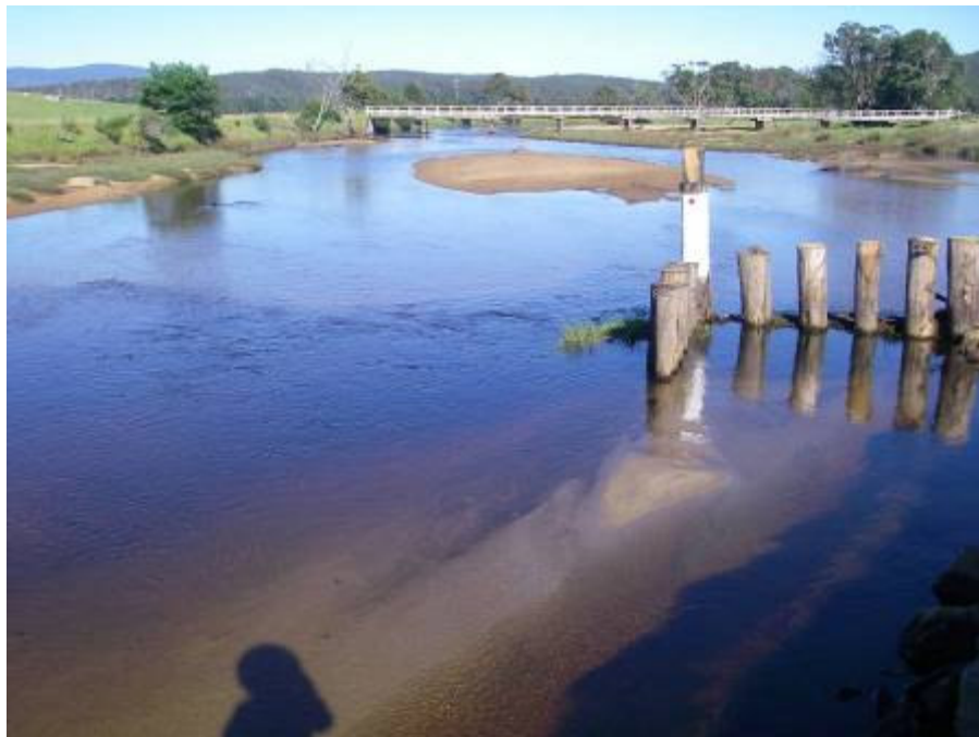
Figure 4b – Pin groyne and scour pool/sand deposit formed following the first bankfull flow event in Feb 08.
