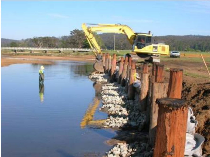
Figure 3 – Log wall construction, Nov 07
