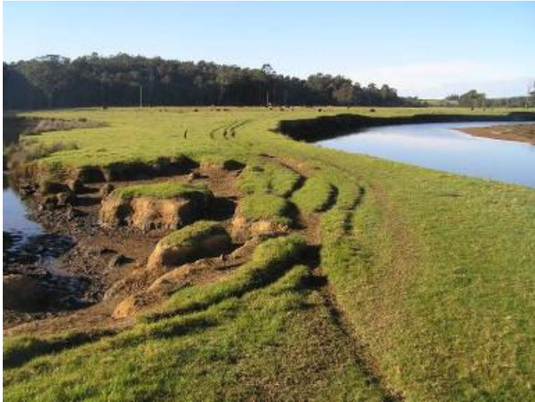
Figure 2 – Photo showing erosion, a lack of riparian vegetation and unrestricted stock access along the Murrah River at commencement of the project – at the narrowest point only 4 m of land remained between the main river (on the right) and the top of a flood channel (to the left).
