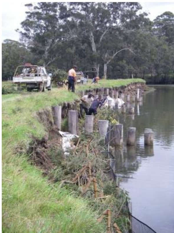
Figure 5 – Brush bundles installed along the toe of the banks, Dec 2008
