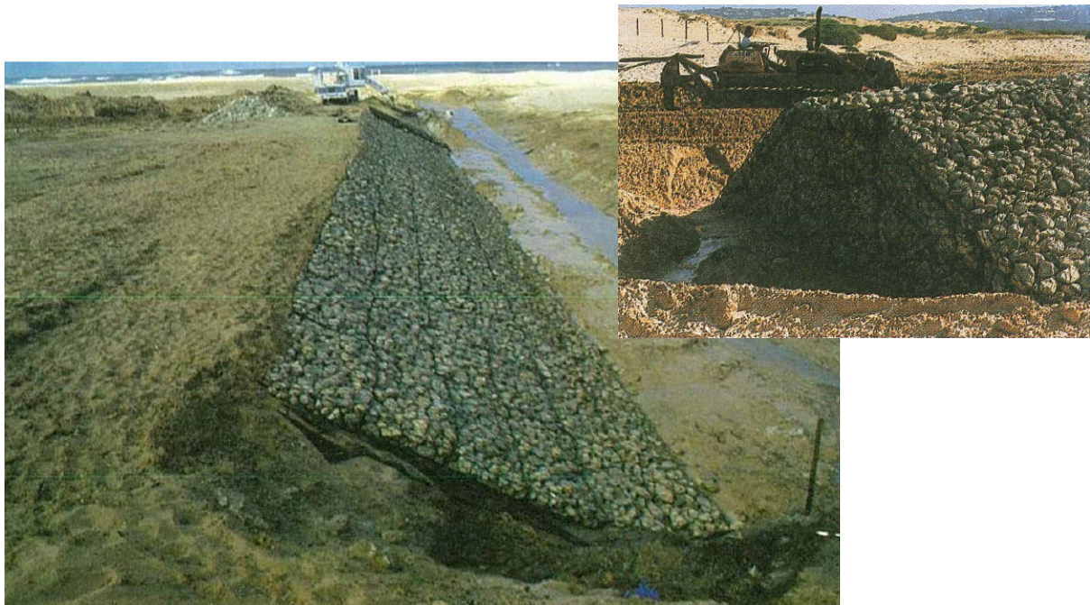
Figure 4: The partial training wall under construction at Dee Why Lagoon entrance (from PWD, 1984). The main photo shows the intent for the training wall to be largely buried.
