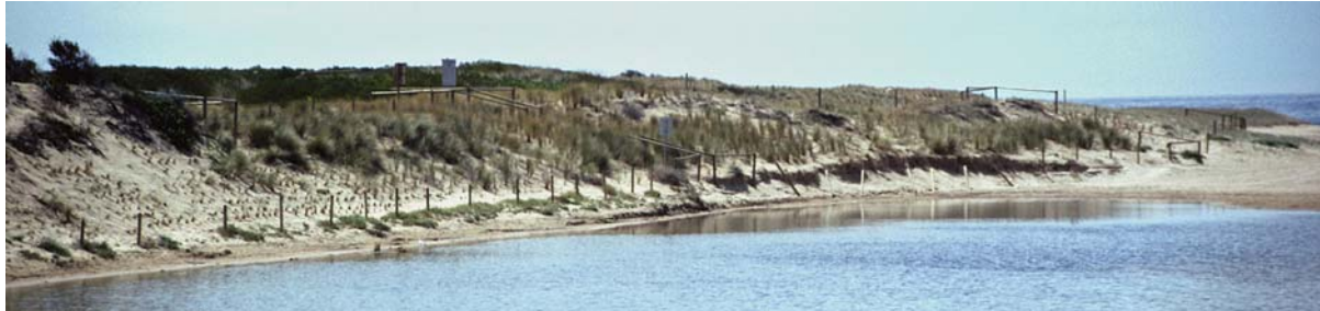
Figure 5: Photo of the completed dune stabilisation works as they looked two years after completion in October 1992. Dune erosion has already occurred and part of the fencing has been undermined.
