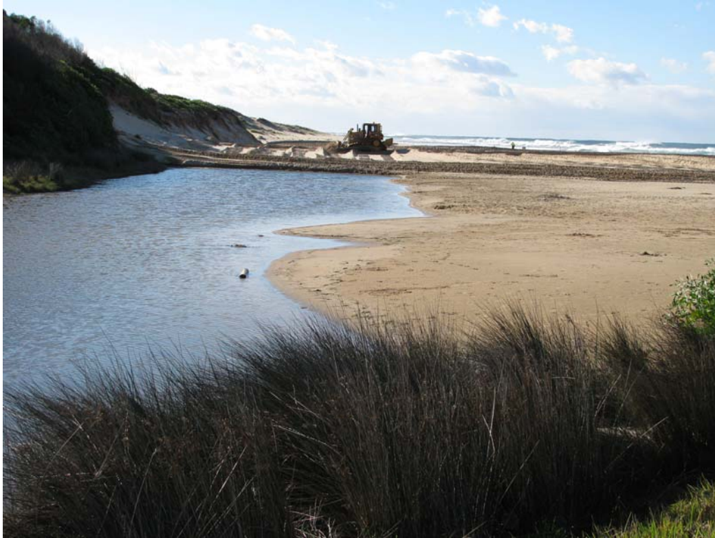
Figure 9: Initial entrance realignment works involving using a bulldozer to infill the northern channel (pictured) and create a pilot channel to the south (taken 10/6/2010).
