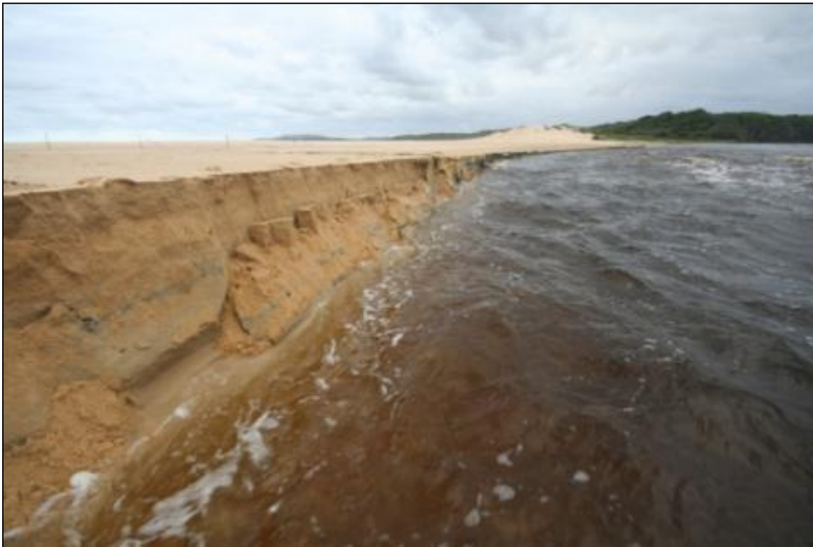
Figure 6 Tabourie Lake 13/02/2008, Breach side walls collapse in shallow slipping failures. The process is small compared to typical cell, element or grid sizes used in numerical modelling and is a challenge to represent reasonably.
