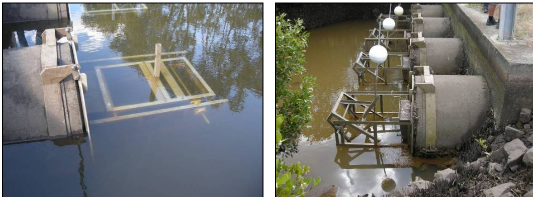
Figure 3. Installed SwingGates in closed (left) and open (right) positions.
