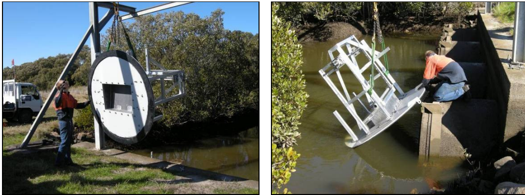
Figure 2. SwingGates being installed
