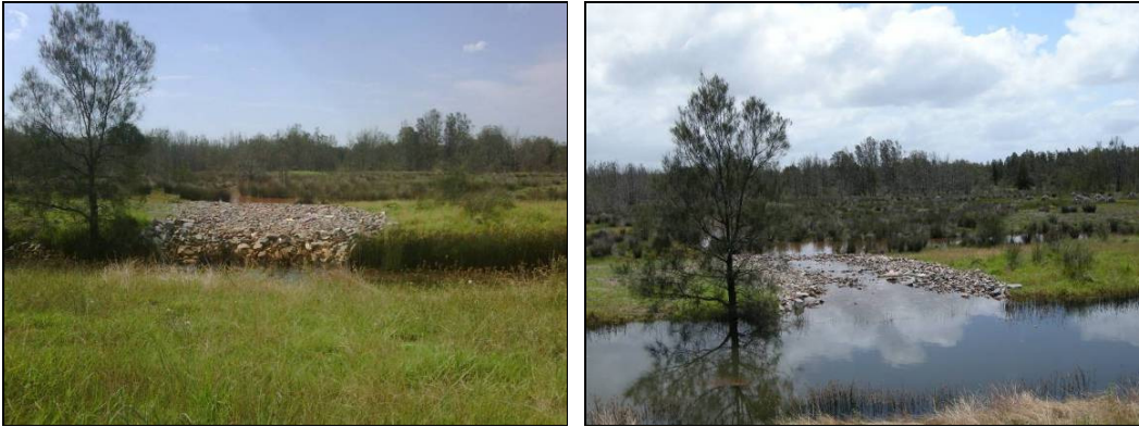
Figure 5. Dish drain at low tide retaining relic drain water levels (left) and reconnecting relic channels at high tide (right)
