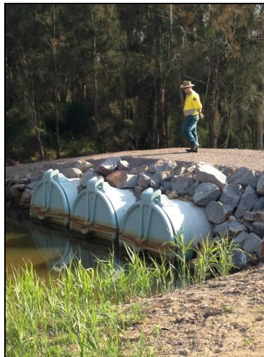
Figure 6. Stage 3 Eastern culverts and floodgates
