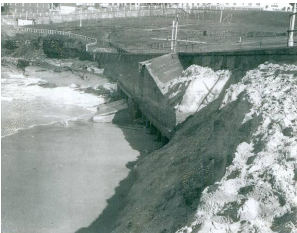
Figure 18: Loss of backfill of mass gravity seawall at South Bondi Beach 13 th June 1974 as a result of toe scour and undermining of the footing (Source Waverley Council; photo by J D Aiosa)
