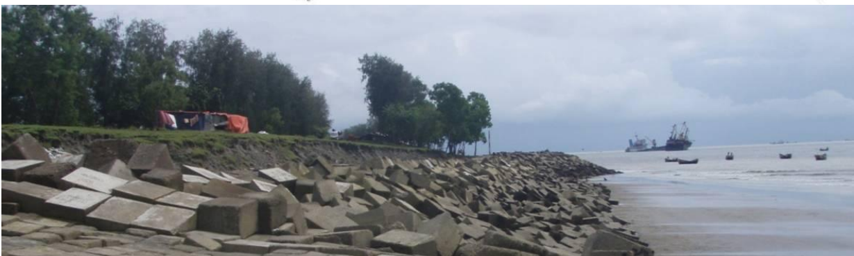
Figure 25: Concrete blockwork revetment failure due to wave overtopping (source Top: USACE 2011; Bottom: Chris Adamantidis)
