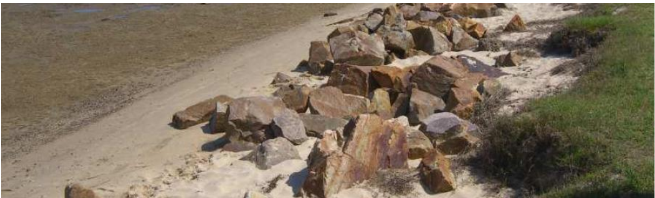
Figure 27: Subsidence of Rock Armour into sand due to inadequate underlayer filtering (source Top: USACE 2011; Right: Chris Adamantidis)
