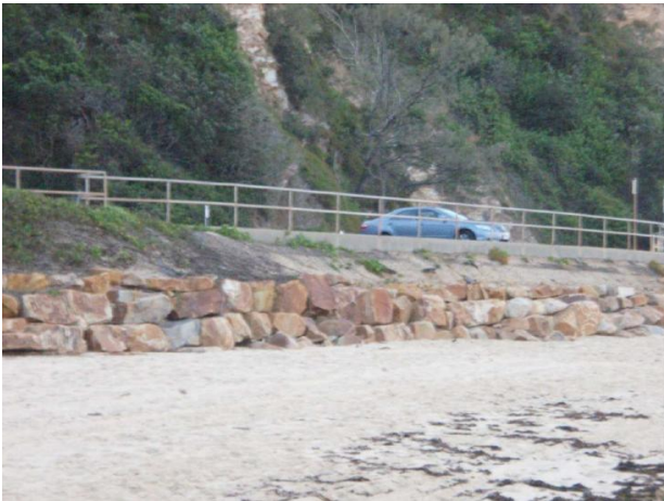
Figure 21: Left: Blockwork Gravity Wall (source Chris Adamantidis); Right: Blockwork Gravity wall failure due to wave overtopping (source Chris Adamantidis)
