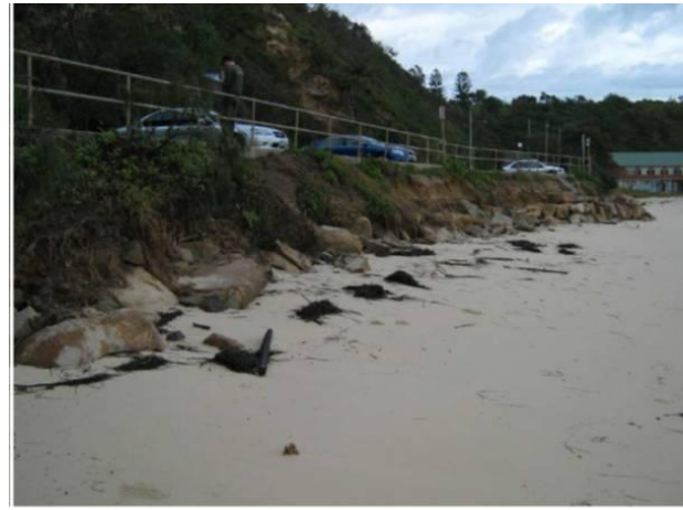
Figure 21: Left: Blockwork Gravity Wall (source Chris Adamantidis); Right: Blockwork Gravity wall failure due to wave overtopping (source Chris Adamantidis)
