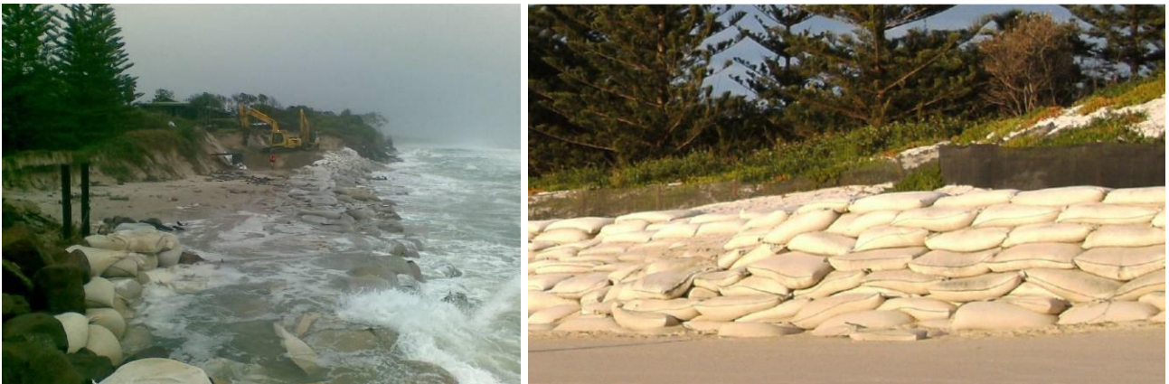
Figure 22: Sandbag seawall failures Left: Pull-out of sand bags due to wave overtopping Right: Pull-out of sand bags due to low frictional properties of geotextile (source Left: Ben Fitzgibbon, Byron Shire Council; Right: Manly Hydraulics Laboratory)
