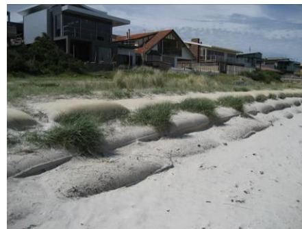
Figure 12: Sandbag revetment (source: Geofabrics Australasia)
