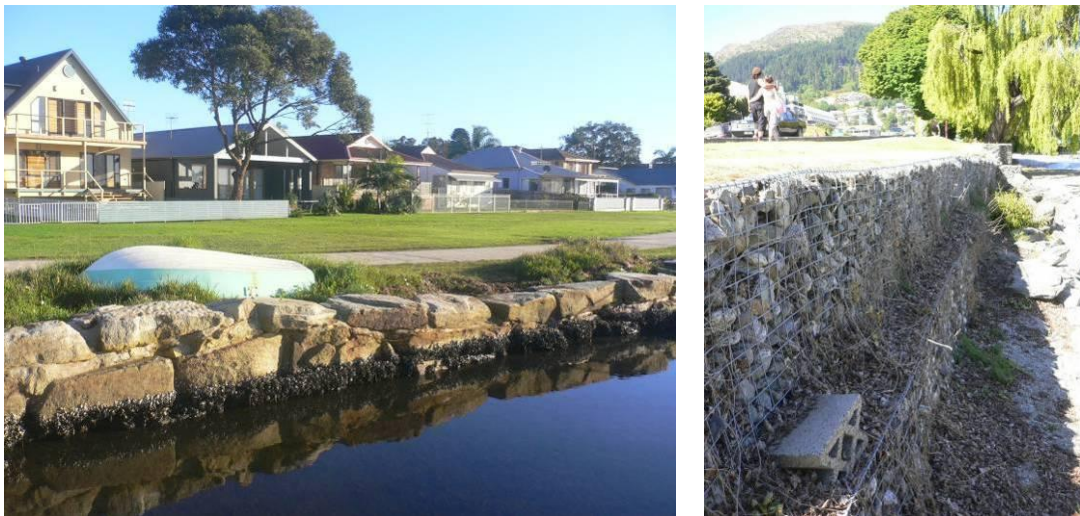
Figure 10: Flexible near-vertical mass gravity seawall Left: Rock boulder gravity seawall (Source Deborah Lam); Right: Gabion gravity seawall (Source Deborah Lam)
