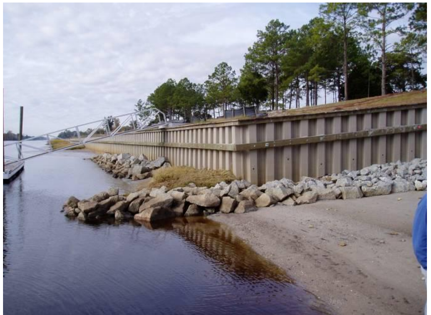
Figure 2: Anchored bulkhead wall
