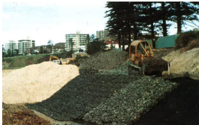
Figure 13: Sloping Reno-mattress dune revetment under construction (Source: NSW Gov., 1990)
