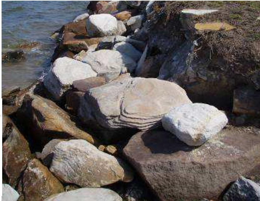
Figure 26: Toe erosion causing subsidence of a boulder wall
