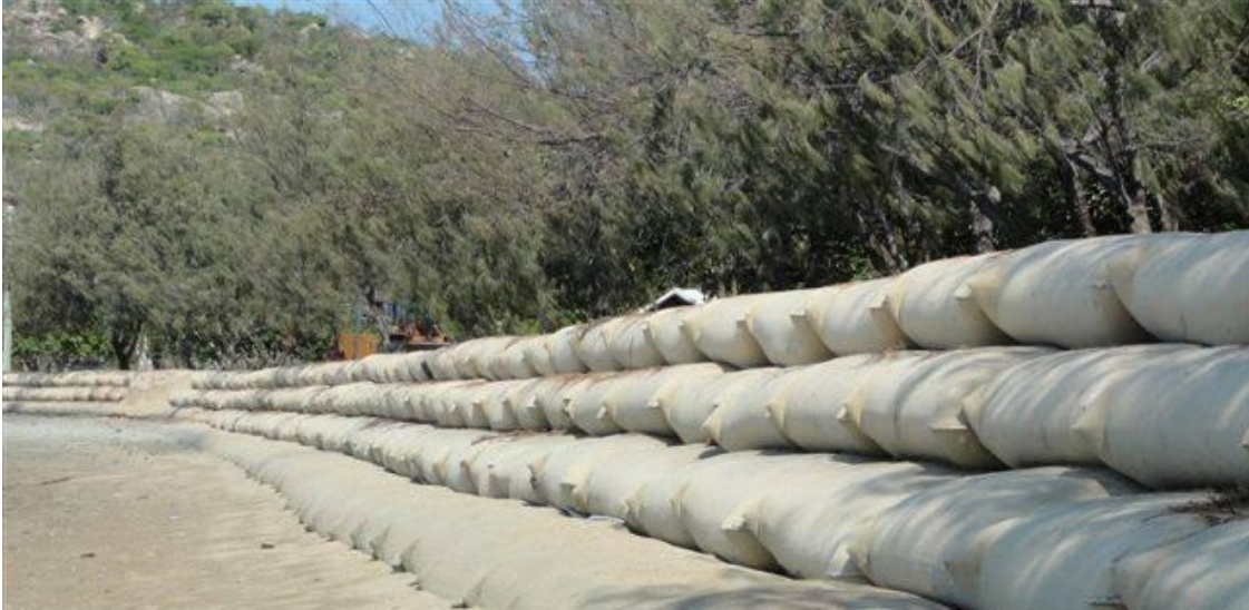
Figure 9: Sandbag gravity seawall (source: Geofabrics Australasia)
