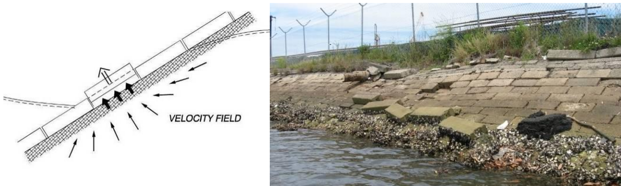
Figure 23: Rigid sloping revetment push-out and subsidence failure modes Left: Push out schema for sloping slab revetments; Right: Subsidence due to incompetent substrata (source Left USACE 2011; Right Tom Pinzone)
