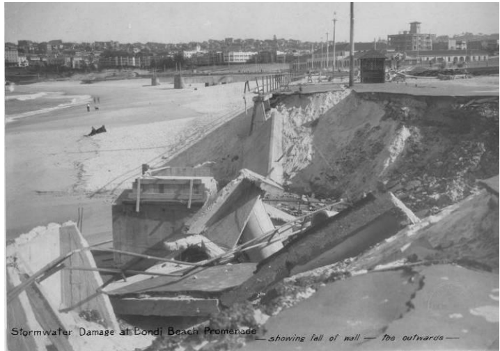
Figure 17: Rotation slip failure of counterfort gravity seawall resulting from toe erosion (source Left: USACE 2011; Right: Waverly Council)
