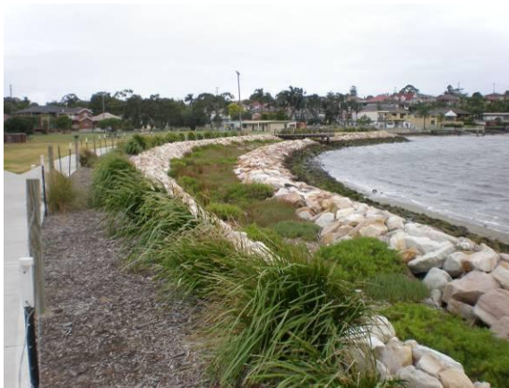
Figure 14: Environmentally friendly seawalls Left: Step-type seawall with saltmarsh (Source WorleyParsons) Right: Estuary bank protection (Source WorleyParsons)
