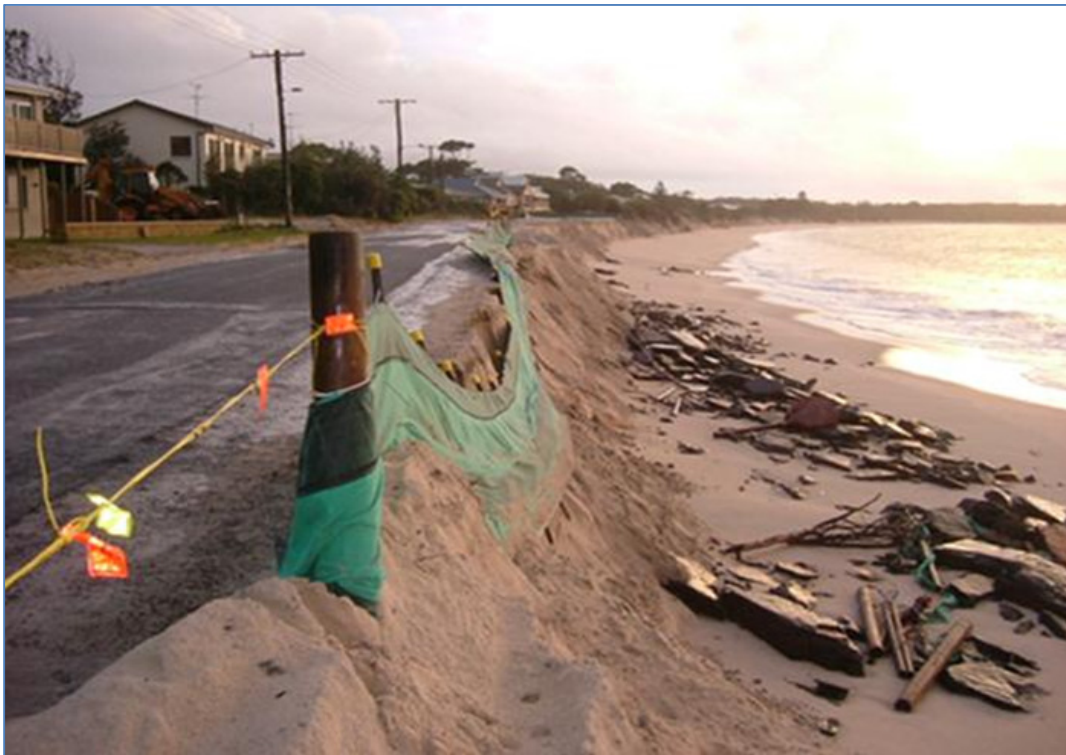
Photograph 4. Existing and future foreshore erosion at Jimmys Beach was the focus of the Great Lakes Council pilot workshops (Source: Great Lakes Council).
