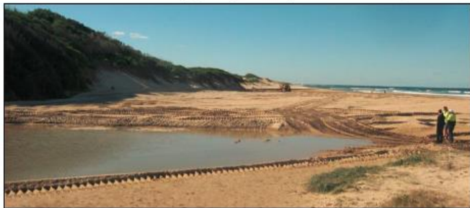
Plate B-2 Beach scraping with excavator in background, June 2010
