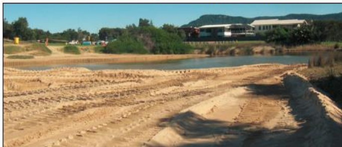
Plate B-3 Beach scraping - safety tape in background at carpark, June 2010
