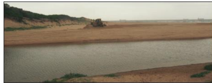
Plate B-4 Beach scraping with excavator on northern side of channel, March 2011
