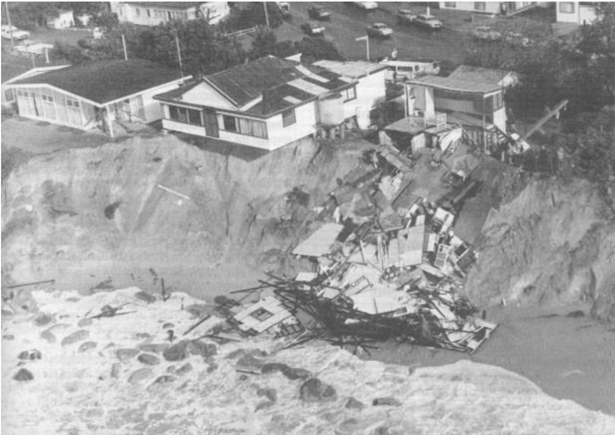
Plate 1 – Beachfront House Collapse – Wamberal 1978 (Photo courtesy: DNR)
