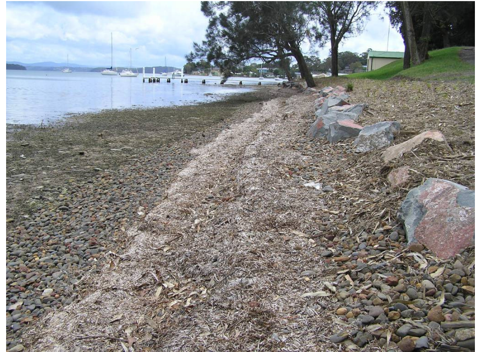
Figure 7 - Nords Wharf Reserve (after). Note return of foreshore slope, protection of toe of bank and seagrass wrack on the cobble beach.
