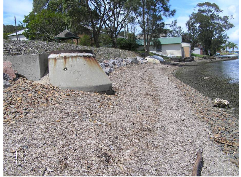
Figure 5 - Wippi Reserve, Coal Point (after). Note foot of bank stabilised with rock, extended foreshore run & accumulation of wrack on foreshore out of the water.
