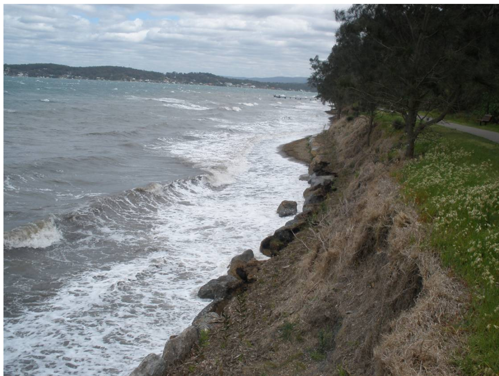
Figure 14 -Green Point foreshore during large storm event. Note change in lake level and waves breaking directly on toe protection rocks.
