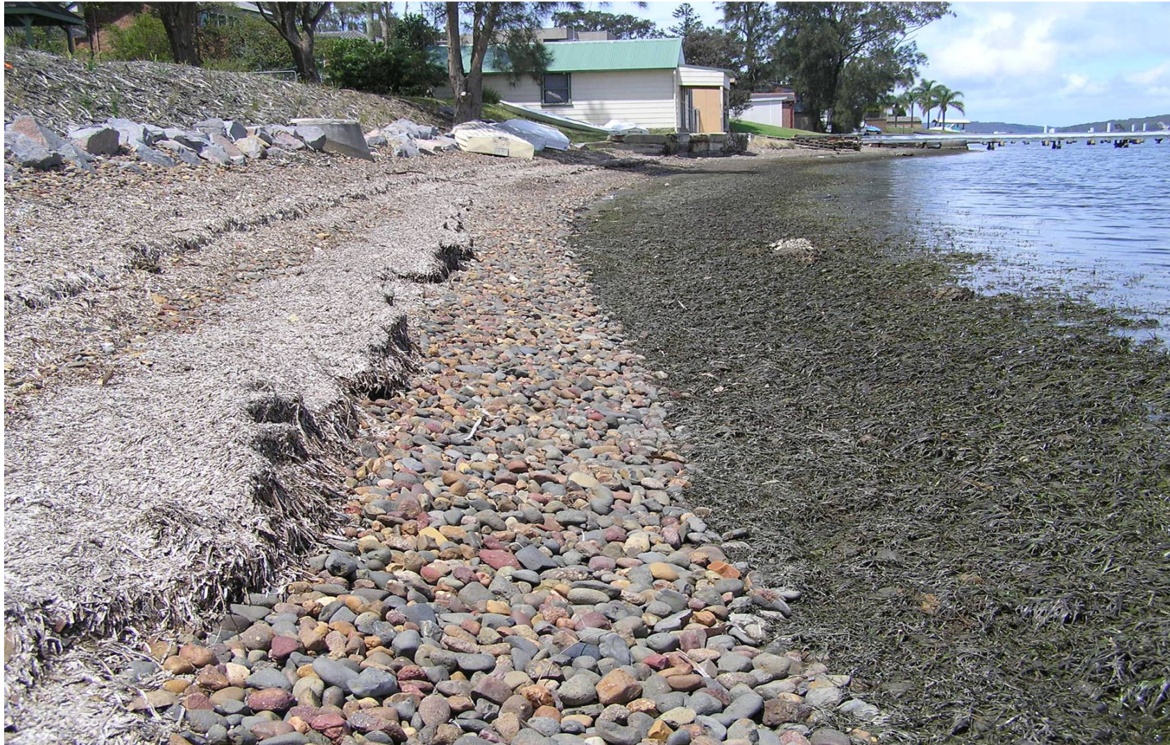
Figure 11 - Side view of Wippi Reserve foreshore profile after restoration. Note the effect the cobble beach has on moving sea grass wrack up the foreshore. Prior to installation of the cobble beach the 'mini-escarpment' would trap the wrack in the Lake water limiting the breakdown of the wrack. The cobble beach has created a zonation of stages of wrack decomposition from the near shore to upper foreshore. (Note this photograph was taken at a time of low lake level exposing sea grass beds usually inundated by Lake water.
