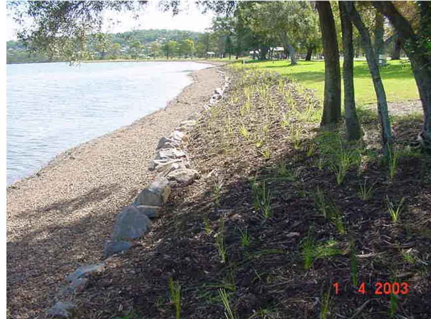
Figure 1 - Speers Point (after). Note sloping beach installation, protection of foreshore bank toe, native plants, and improved amenity.
