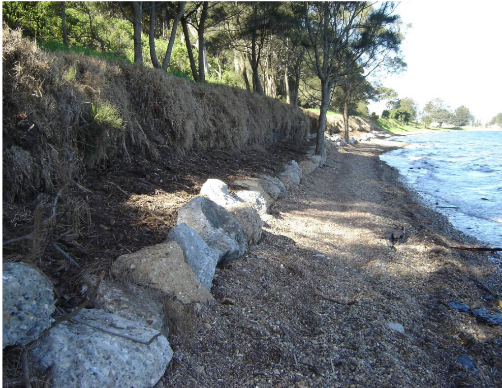
Figure 13 - Green Point foreshore (after). Note installation of toe protection.
