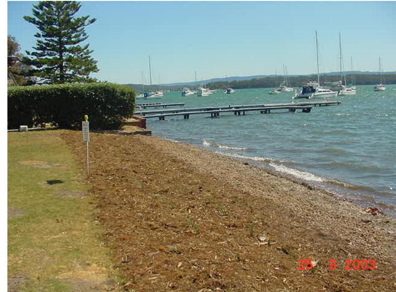
Figure 3 - Valentine foreshore (after). Note improved foreshore slope angle designed to facilitate wave energy dissipation to prevent 'mini-escarpment' development.
