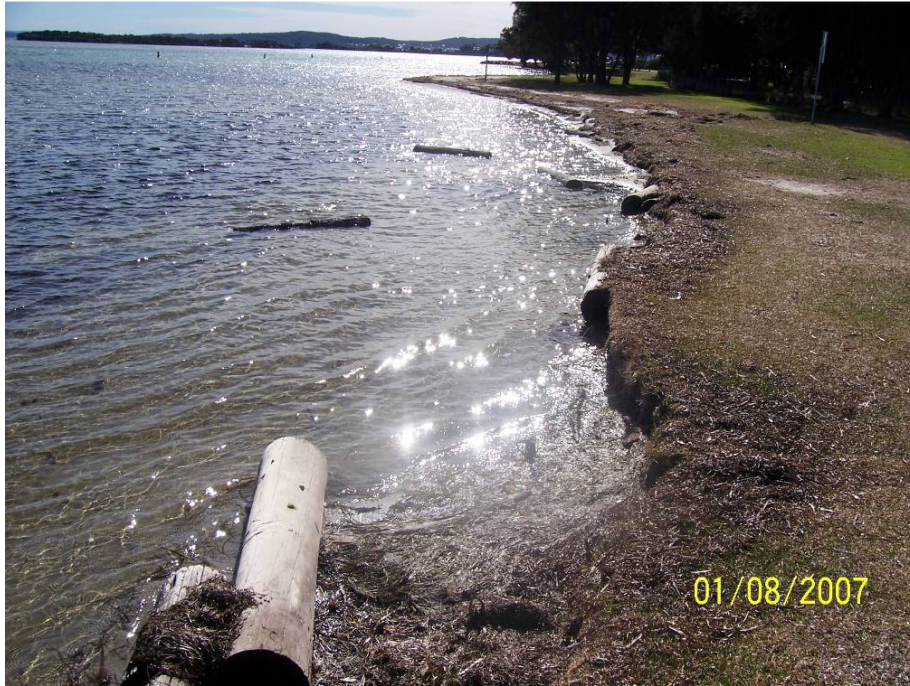
Figure 10 - Swansea Channel (before). Note 'mini-escarpment' along foreshore edge, accumulation of sea grass and failing foreshore revetment (logs).
