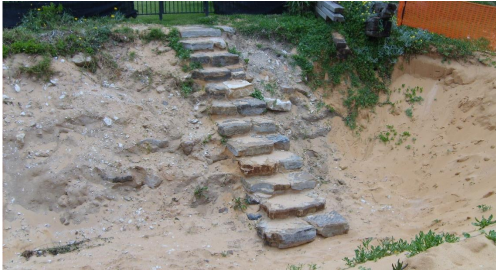
Figure 3: View after initial removal of illegal seawall, November 2011
