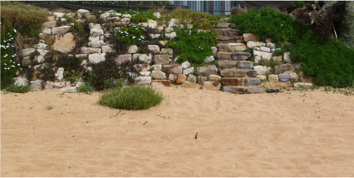
Figure 1: Illegal seawall about 2 years after construction, in March 2010
