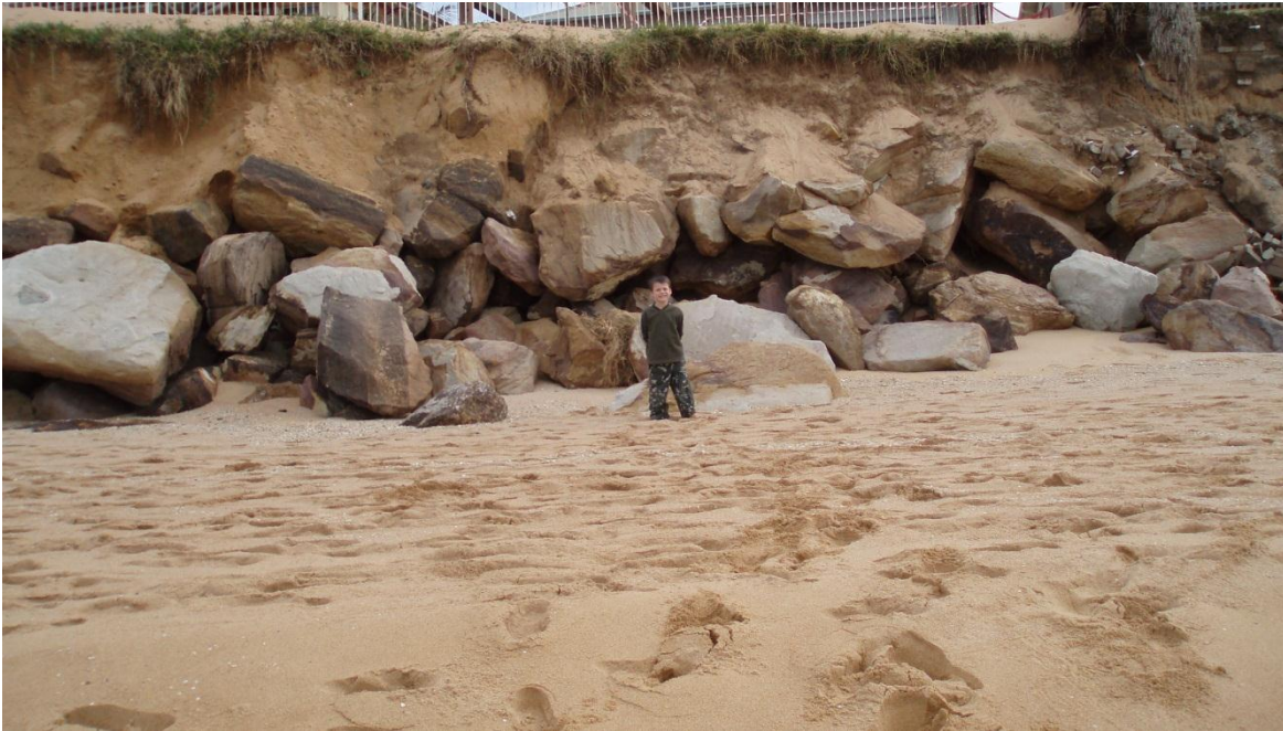
Figure 2: Historical protection works exposed at subject property in July 2007
