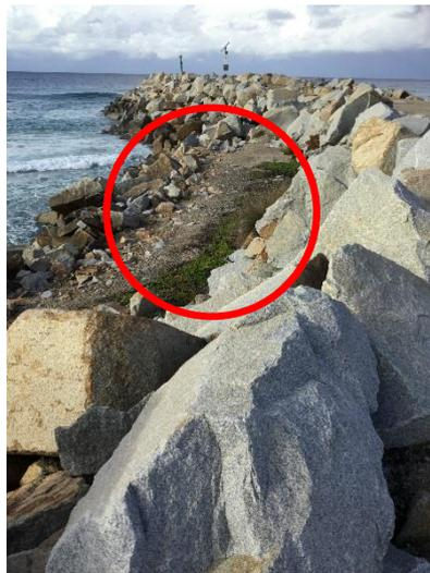
**Figure 11 Relatively minor (<2%) damage to Narooma north training wall crest (in comparison with Moruya north) possibly due to unique berm construction on ocean side**
