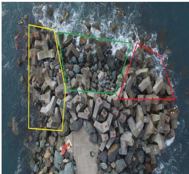
**Figure 8b Forster training wall – extensive head damage post-2016 storm**
