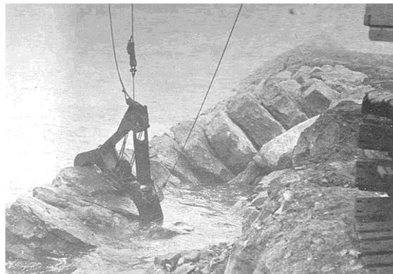
Figure 12b Special placement  $K_d = 4-8$  (CERC)
