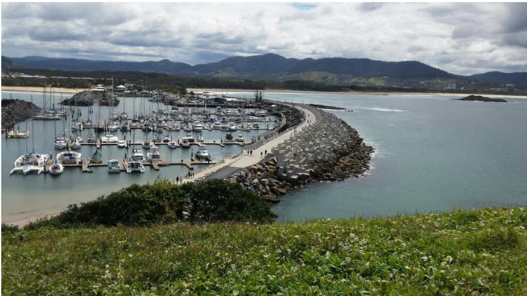
**Figure 6c** Completed breakwater showing 5m berm of 5–8t rock overlain by 12t Hanbars with 2 x 20t Hanbars as containment on seaward side
