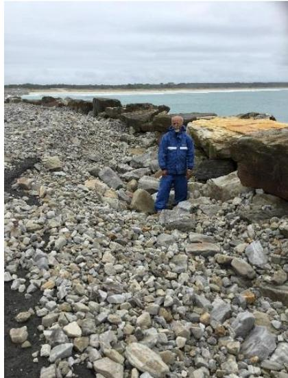
**Figure 5c Clarence north training wall crest post-June 2016 storm – closer view of crest damage**
