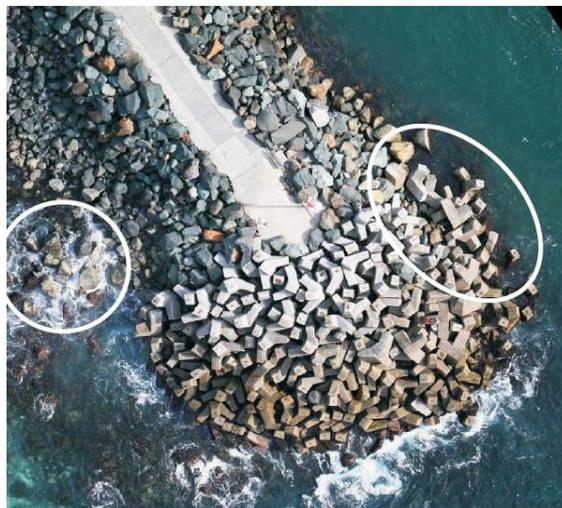
**Figure 8a Forster head damage after 1-in-40-year ARI storm in 2009**
