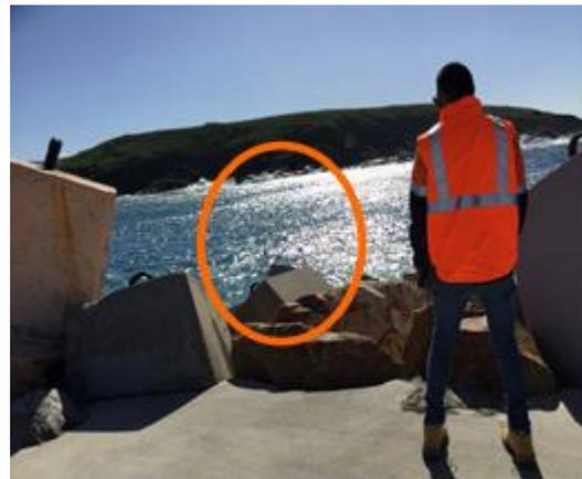
**Figures 10c and 10d Relatively minor (<2%) damage to Coffs Harbour east breakwater head after June 2016 storm**
