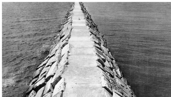
Figure 12c Special placement  $K_d = 8-10$  (CERC)
