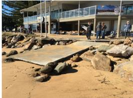
Foreshore erosion and damage to inadequately designed (ad hoc) structures
