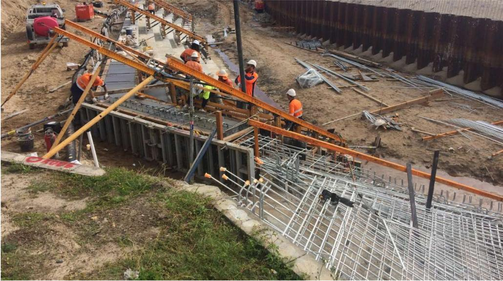
Placement of reinforcing steel and pouring of the lower portion of the structure
