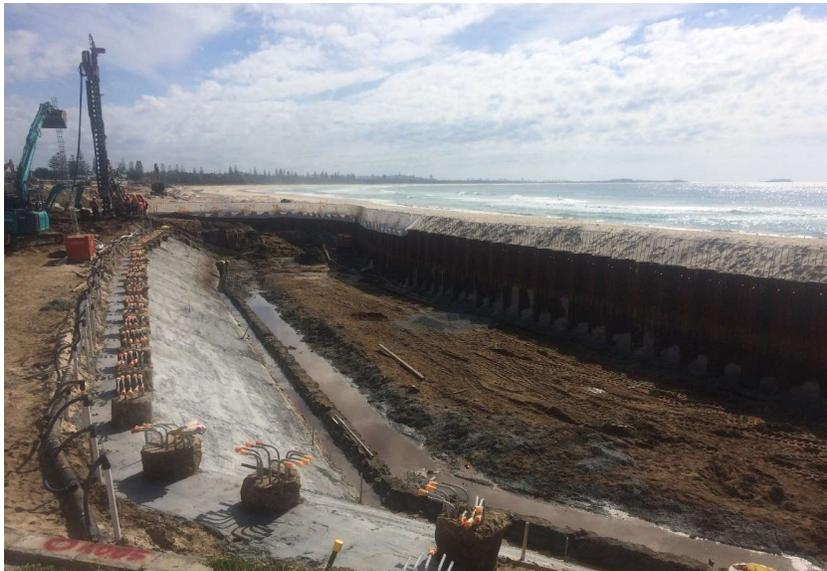
Lower secant wall and upper piles with blinding layer installed
