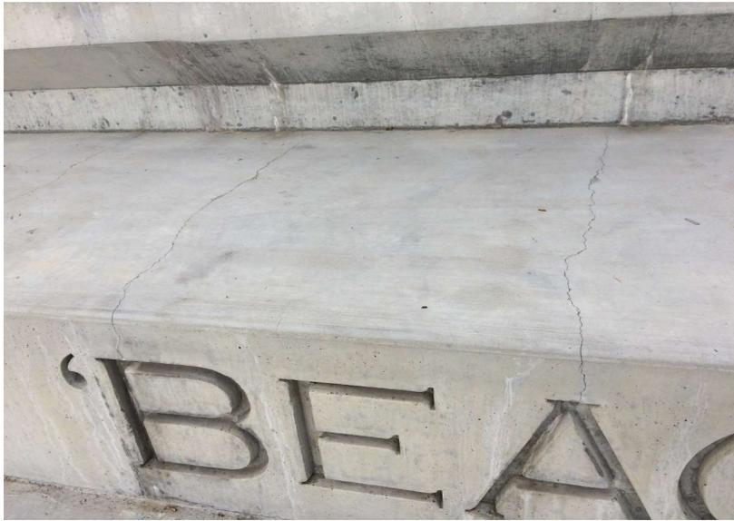
Early cracking of the concrete seawall structure, specifically the upper portion
