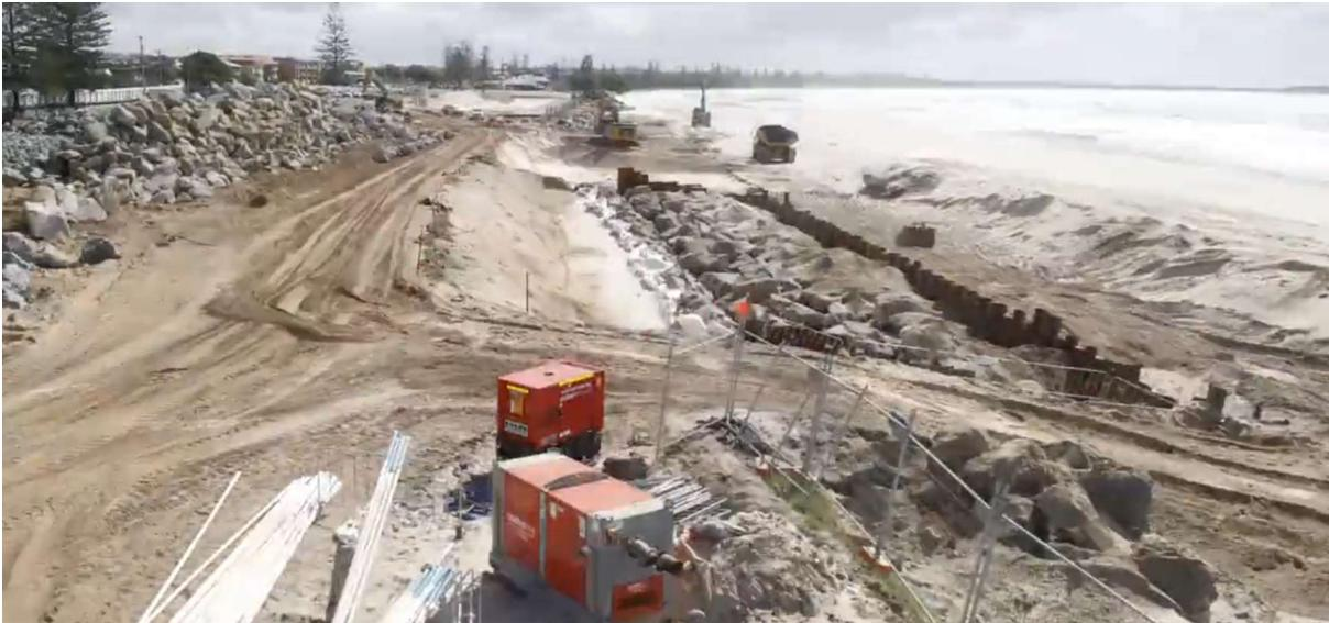
Excavated material used to backfill to existing beach level, second cofferdam being prepared in the background
