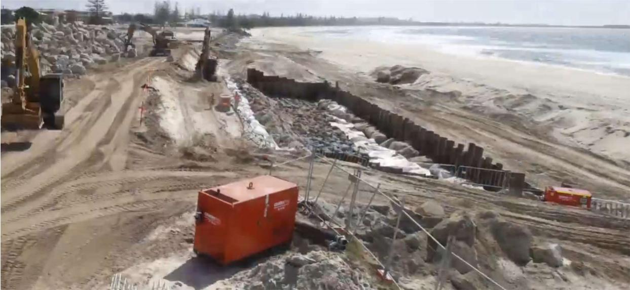
Work continues in the dry with the placement of geotextile and filter rock
