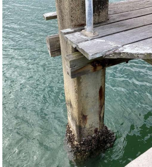
Cracking and reinforcement corrosion leading to spalling on unrelated concrete piles
