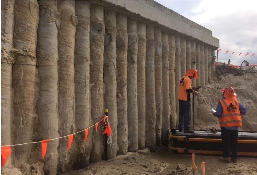
Extent of piling for stepped concrete seawall to abut the existing SLSC structure
