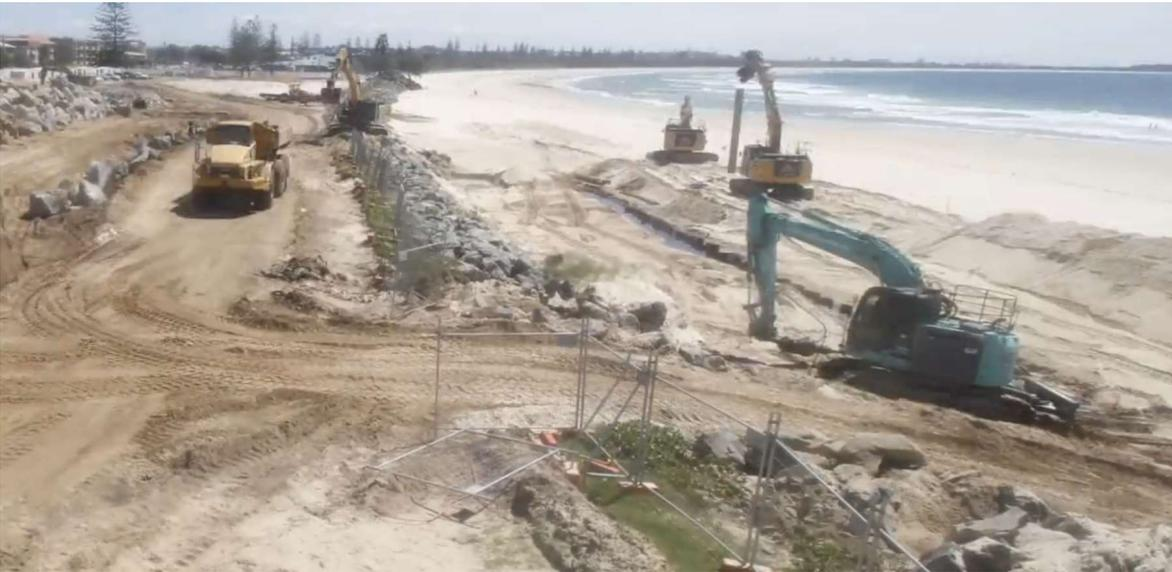
Installation of cofferdam for construction of seawall toe
