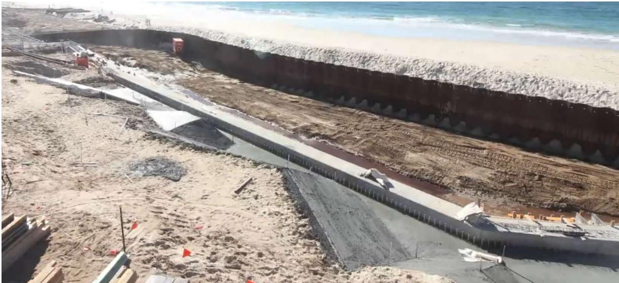
Shaping and blinding of the upper concrete structure
