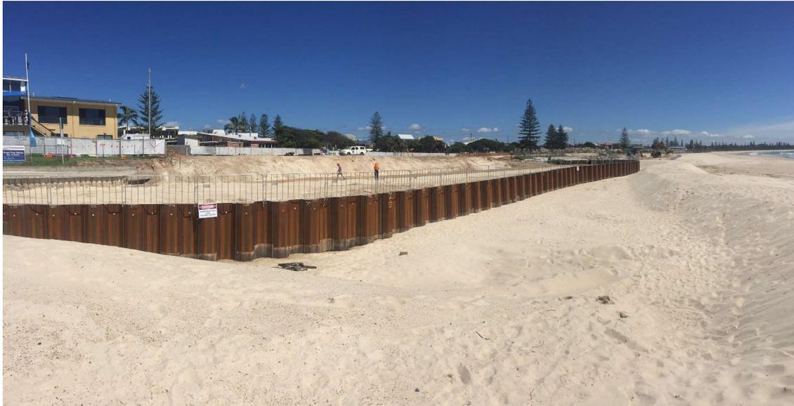
Cofferdam to facilitate construction of the entirety of the stepped concrete seawall
