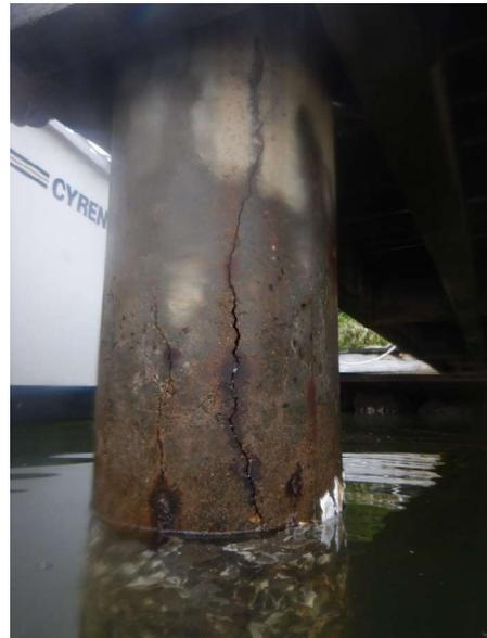
Cracking and reinforcement corrosion on unrelated concrete piles
