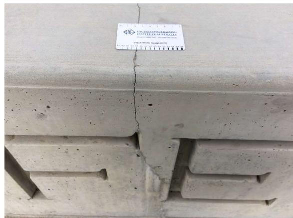
Early cracking of the concrete seawall structure, specifically the upper portion
