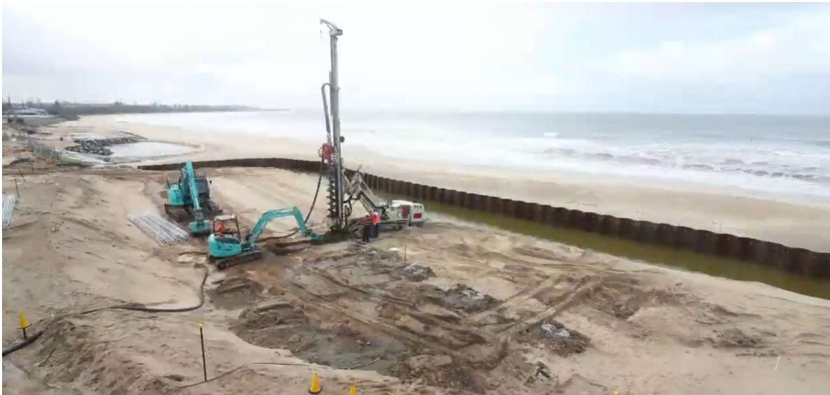
Installation of the pile which will support the upper extents of the lower structure
